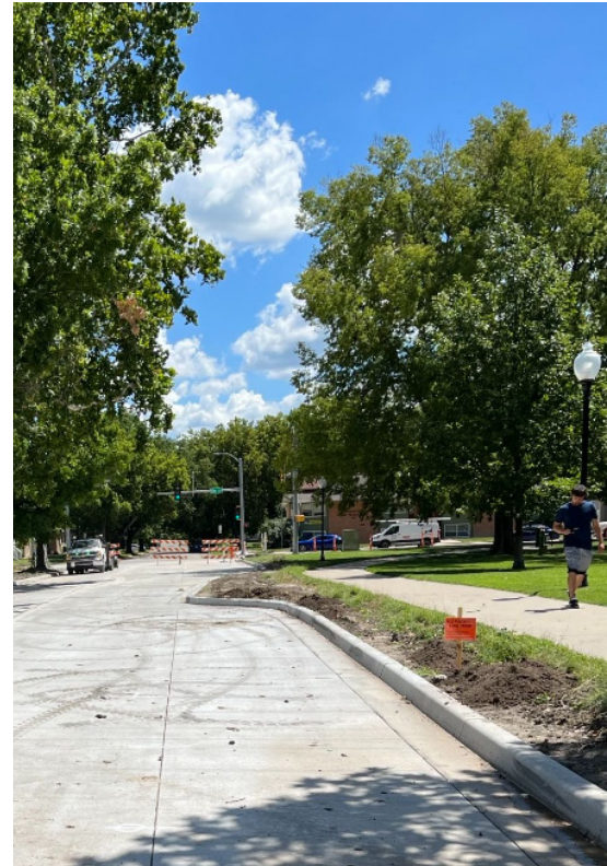
Phase 1 completed with curb extensions.
