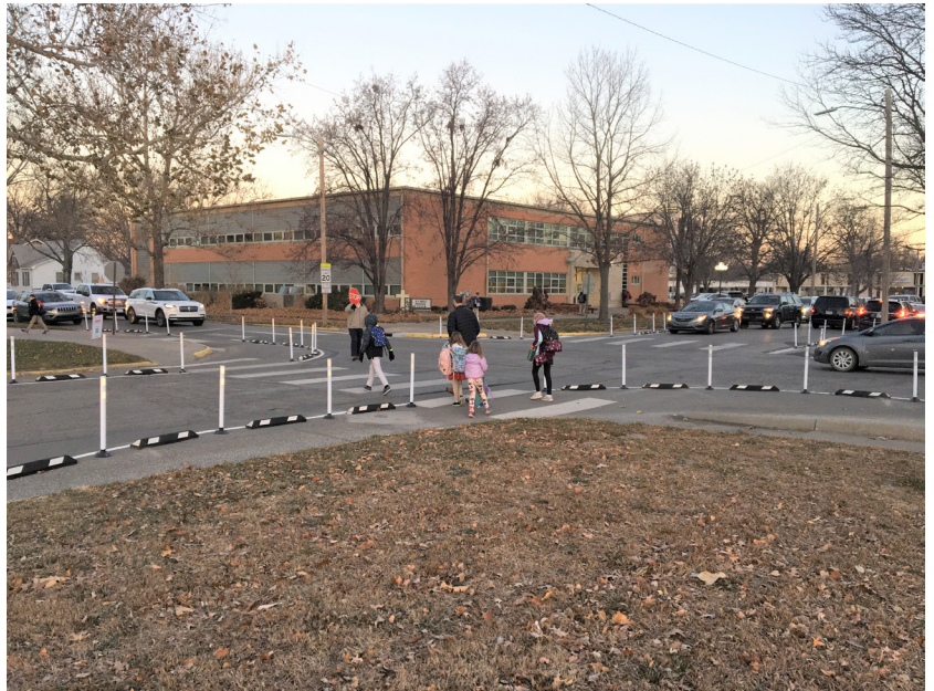
Concrete curb extensions will replace this semi-permanent project one
