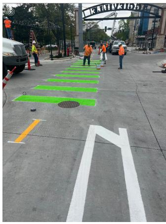
Reconstruct utilities & roadway, new Aggieville streetscape, and 2-way bike lane. Protected at the intersection with Bluemont, this buffered bike lane extends south to Fremont St. Here it will tie into the Fremont St. Improvement project (C4).
